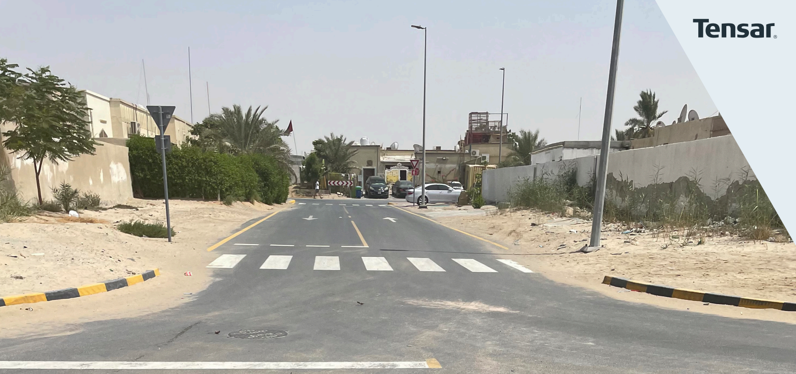
Completed road open for traffic
