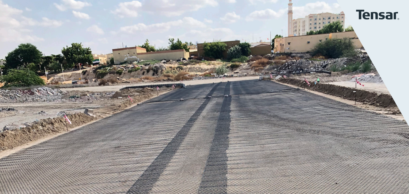
Installation of Tensar geogrids during construction of a Tensar Mechanically Stabilised Layer (MSL)
